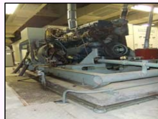
[自家発電設備]
