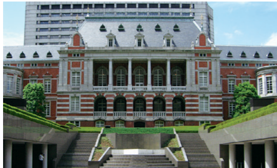
The red-brick building seen from the Sunken Plaza
