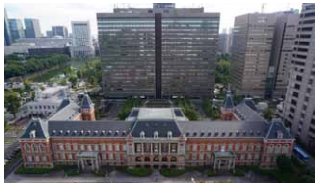
Red-Brick Building and Central Government Office No.6-A
