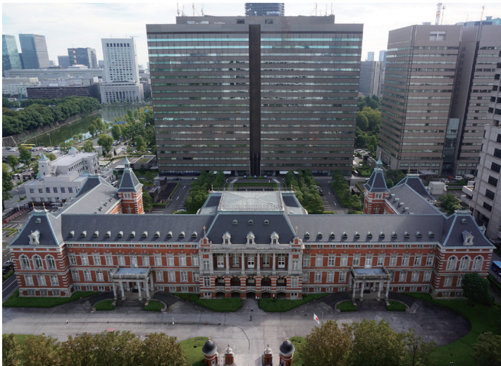
Red-Brick Building and Central Government Office No.6-A
