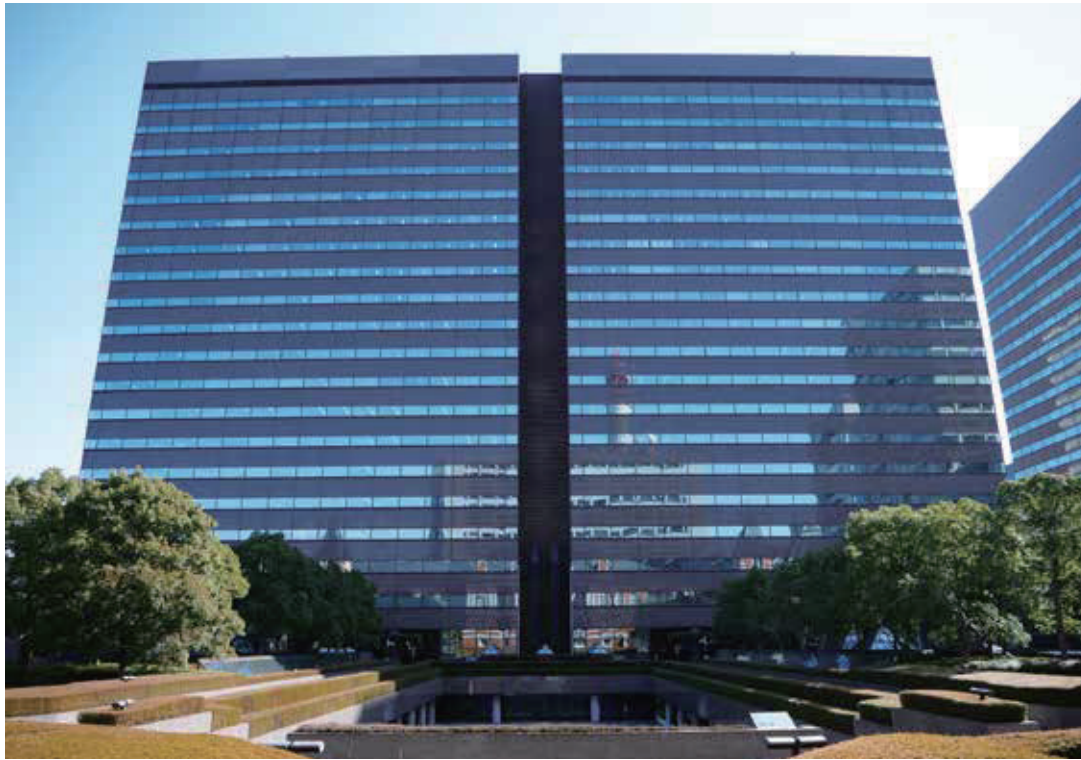
Central Gov't Bldg. No.6
