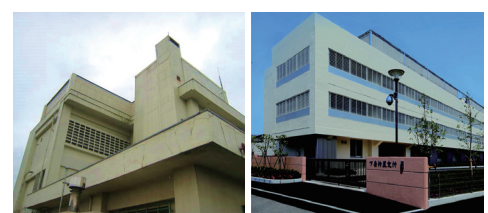
Before life prolongation renovation of Shimotsuma Detention Center (left) and after renovation (right)
