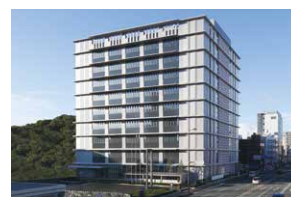
Office building (Tokushima Ministry of Justice office complex)
