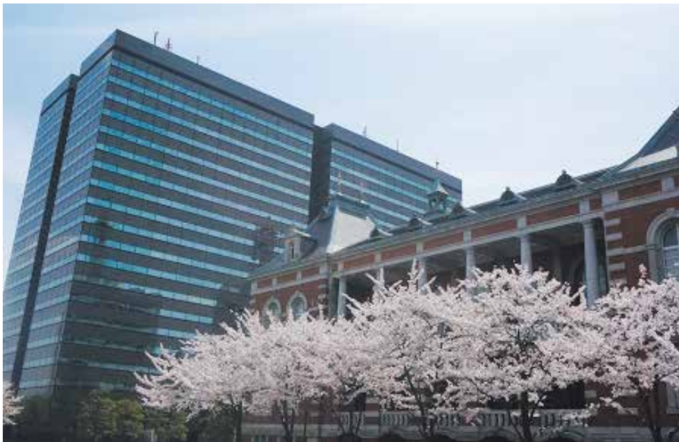
The former and current Ministry of Justice buildings in spring
